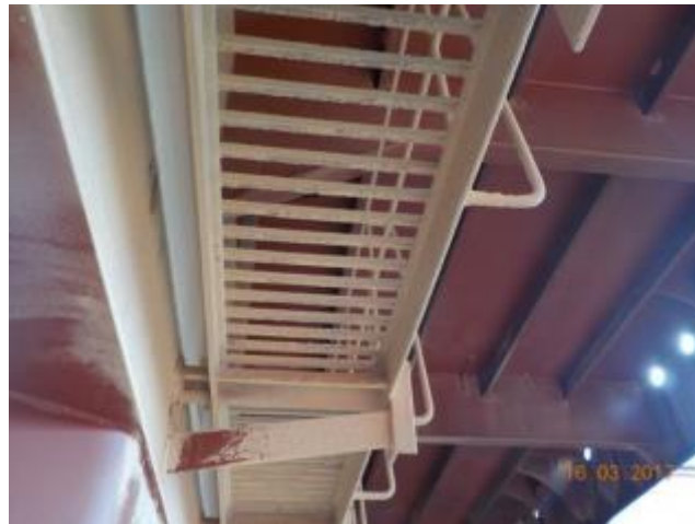
AFT UNDERDECK PLATFORM WITH SBM RESIDUES
