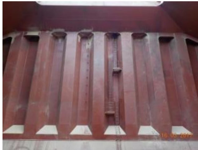
FWD BULKHEAD WITH COAL STAINS
