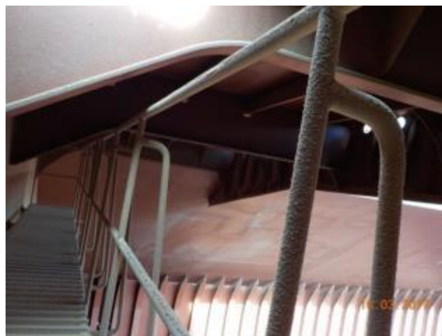
FWD UNDERDECK PLATFORM WITH SBM RESIDUES
